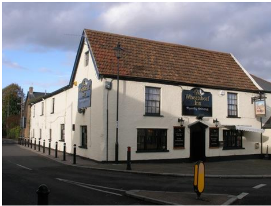
Fig.68 The Wheatsheaf Inn. The low ceilings on the ground floor, steep roof with gable ends and long rear range indicate a building of perhaps 17 th century origins, despite its loss of chimneys and the later windows.
