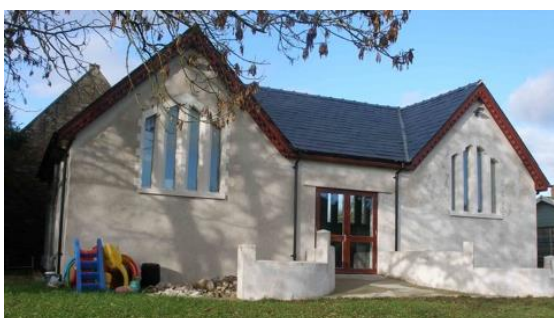
Fig.84 The recent extension of the former School on its south side, in a garden location. The form and some of the detailing respond to the character of the original building.
