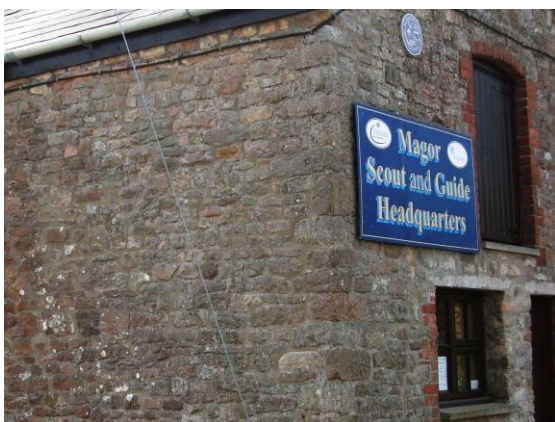
Fig.86 Rubblestone in combination with red brick dressings on the Scout Hall
