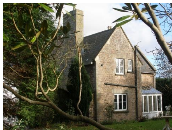
Fig.80 Former School House. A High Victorian design with massive chimneys, tall gables and well executed stonework.
