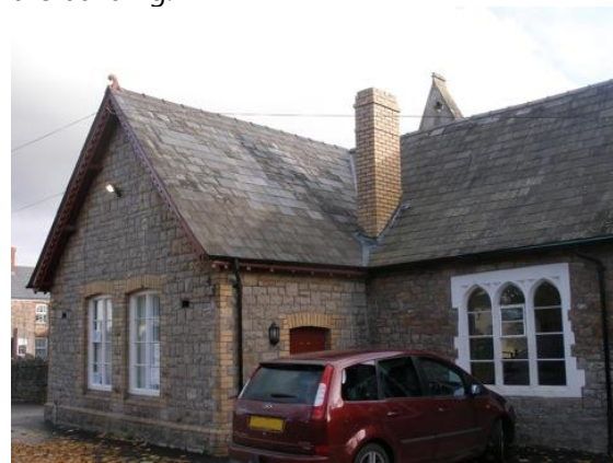
Fig.79 Attached to the School House and designed at the same time, the former School has a belfry, large mullioned windows and a robust design reflecting its function.
