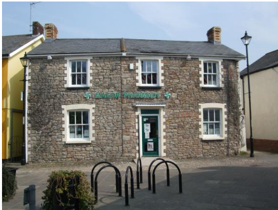
Fig.12 The pharmacy is constructed in rubblestone, one of a number of traditional local materials seen in this part of the Conservation Area
