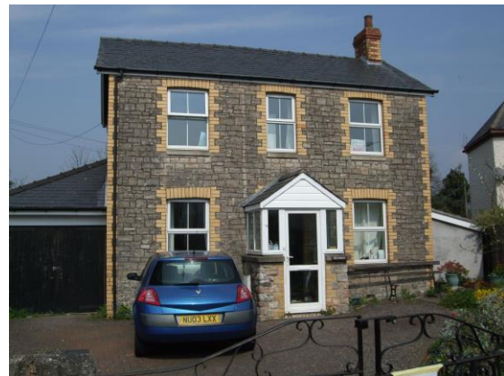
Fig.87 A striking combination of stone with yellow brick dressings, Devonia
