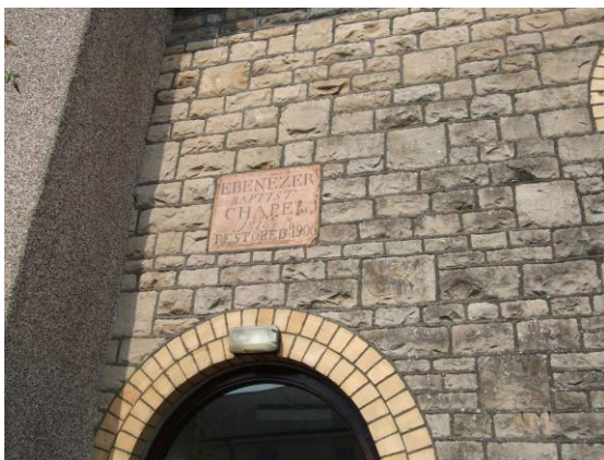
Fig.13 The attractive use of squared stone to the Baptist Chapel used in conjunction with yellow brick dressings
