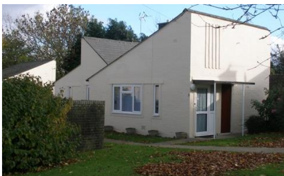
Fig.83 Chestnut Close. Characteristic 1970s houses with monopitched roofs, grouped to create green spaces.
