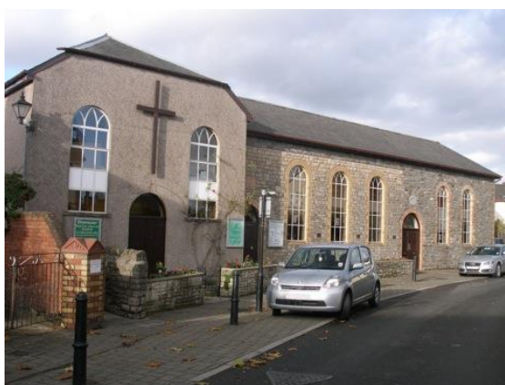
Fig.76 Built in 1816 and subsequently enlarged, the Baptist Chapel retains its characteristic tall window design, although the glazing bars have been replaced.
