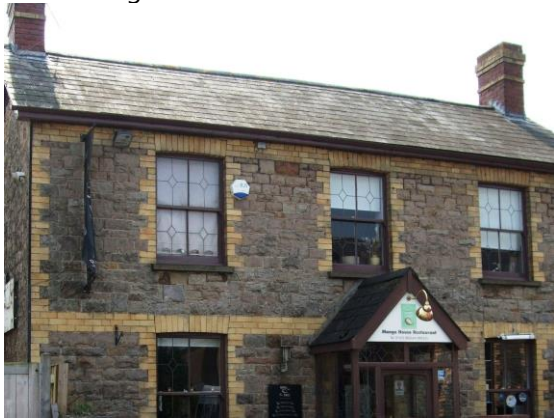
Fig.89 Natural slate is a typical roofing material seen in the Conservation Area
