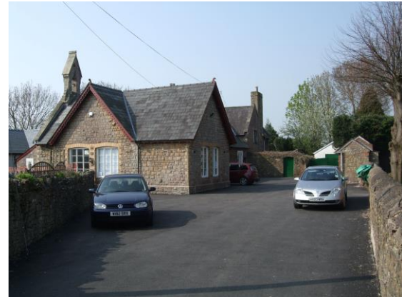
Fig.25 The church school positioned south of the church.
