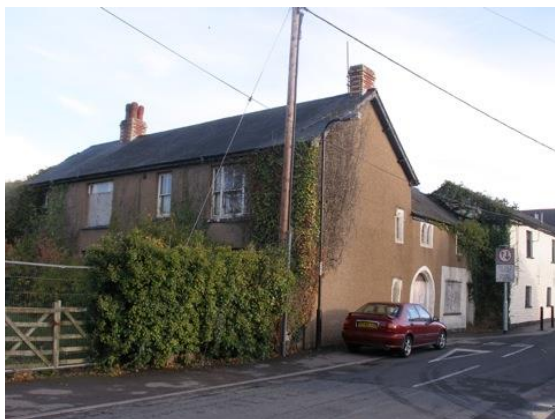
Fig.62 Manor Farmhouse. This vacant farmhouse and associated outbuildings, mainly 19 th century in appearance, incorporates a much earlier side wing.
