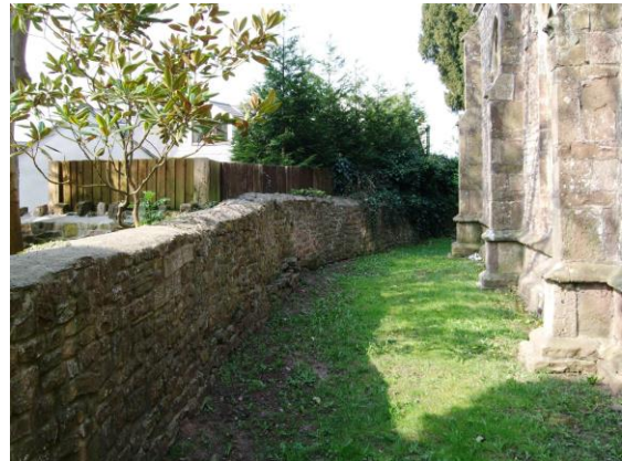
Fig.90 Rubblestone boundary walls strongly define some areas within the town including the churchyard
