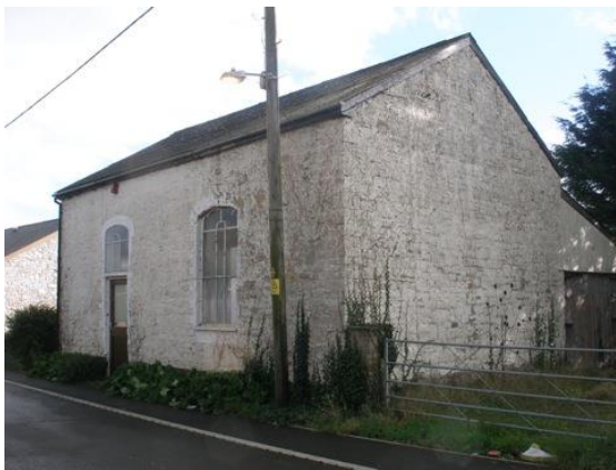
Fig.77 Former Chapel, West End. This vacant building, although extended and in need of sensitive conservation, is a physical reminder of the heritage of Magor, for both its original purpose and simple design.
